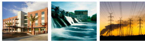
Holding cum Generation cum Transmission Company
